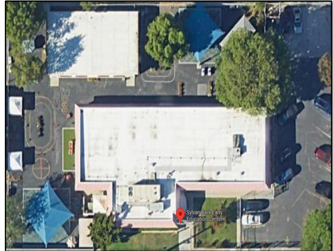
Site Aerial View
